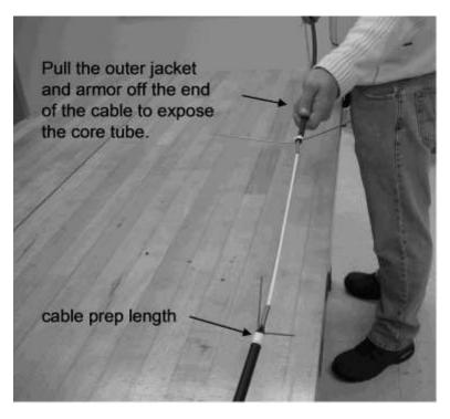
Figure 15 – Remove the outer jacket and armor to expose the core tube.
