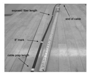
Figure 12- Mark the required cable prep lengths.
