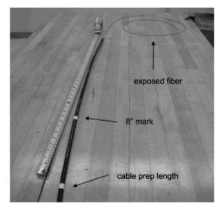
Figure 13 – Remove the outer jacket, armor, and buffer tube to expose the fibers.
