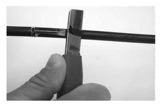
Figure 3 – Shave the cable jacket to expose the strength members.
