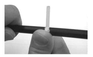
Figure 2- Ring cut the cable jacket.
